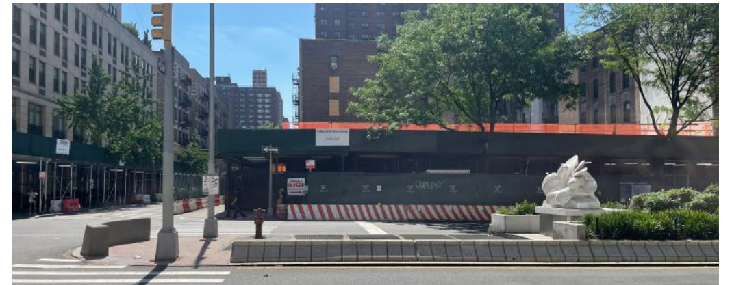
103rd St. Plaza, Looking East
